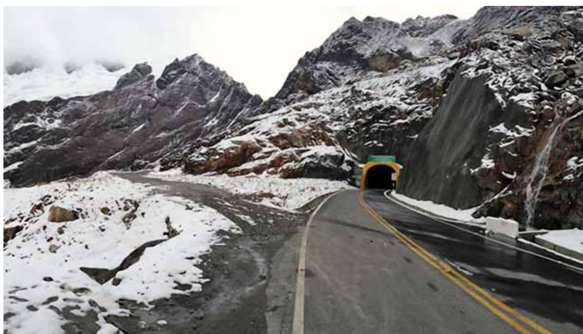
The Olympic tunnel in the Cordilleras, which was inaugurated in 2013. At 4735 metres above sea level it is the highest tunnel in the world. The first tunnel was opened in 1984, but soon had to be closed again because of the danger of avalanches and falling rocks.
